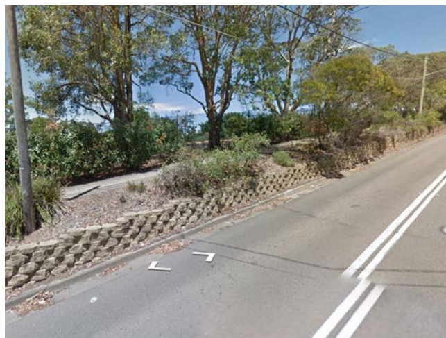
Figure 23: Retaining wall on verge
