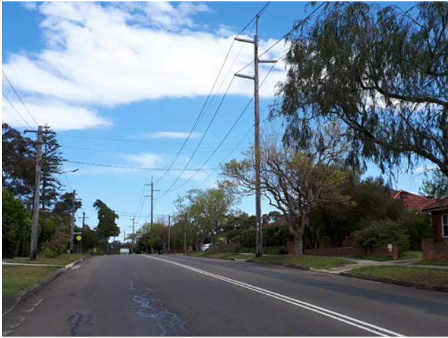
Figure 26: Existing overhead wires
