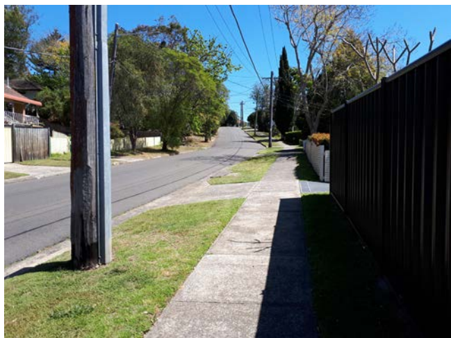
Figure 20: Existing utility poles
