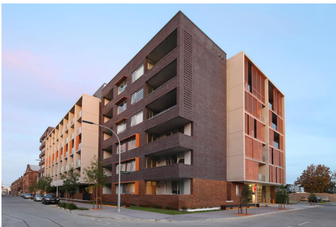
The Platform Apartments Source: Richard Crooke Constructions
