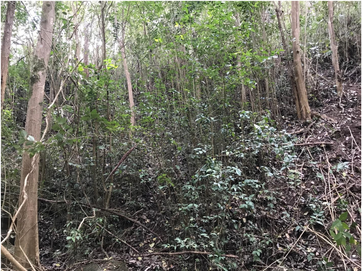
PP04 – MZ1 – Looking north from up slope. Unstable soils within impact area.
