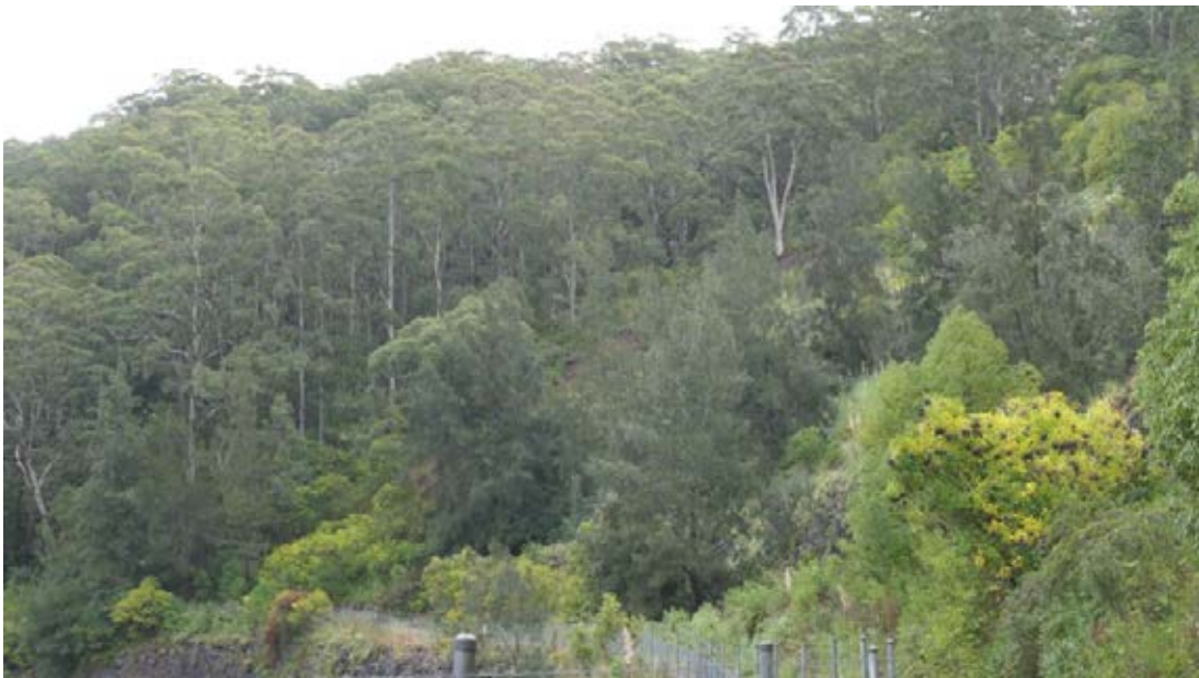
Figure 9 – Northern fill slopes - at right and view to western edge of the fill slope and its interface with the more natural vegetation of the Blue Gum and Blackbutt Gully Forest beyond. (Photo: Arterra 25/7/19)
