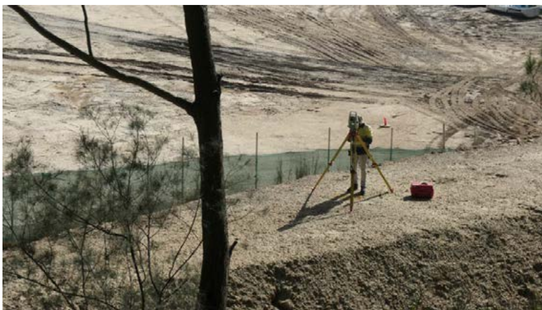
Figure 13 – Photo illustrating that the trees were surveyed using a registered surveyor to accurately position the trees spatially on the site. This was done at the same time as the trees were surveyed and identified by the arborist to maintain consistency, accuracy of recording and numbering throughout. (Photo: Arterra 22/7/19)
