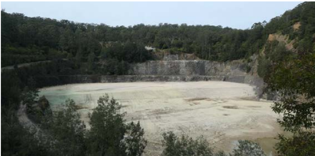
Figure 1 – View from the western side of the now abandoned Hornsby Quarry looking east towards Old Mans Valley. (Photo: Arterra 25 July 2019)
