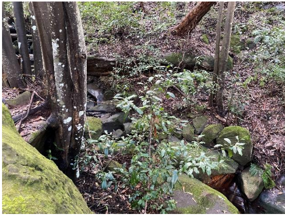
Figure 5: Byles Creek tributary near end of Azalea Grove, looking upstream
