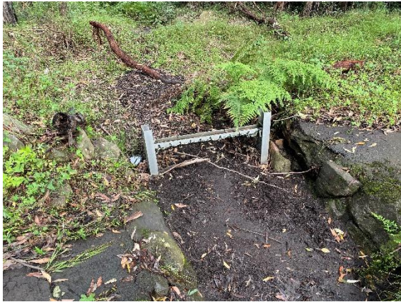
Figure 11: Full gross pollutant trap below Britannia Street
