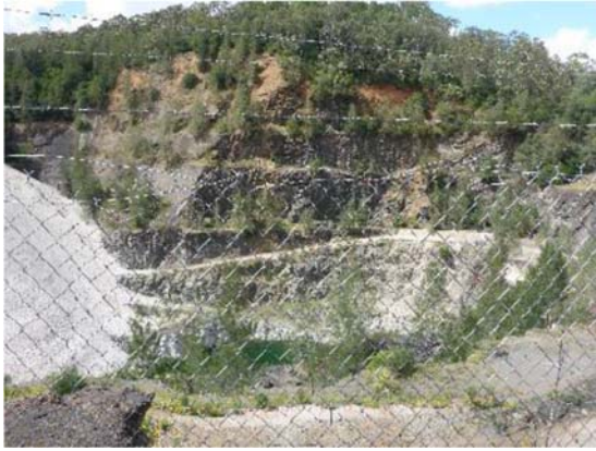
Photograph 12.3 View south of the quarry
