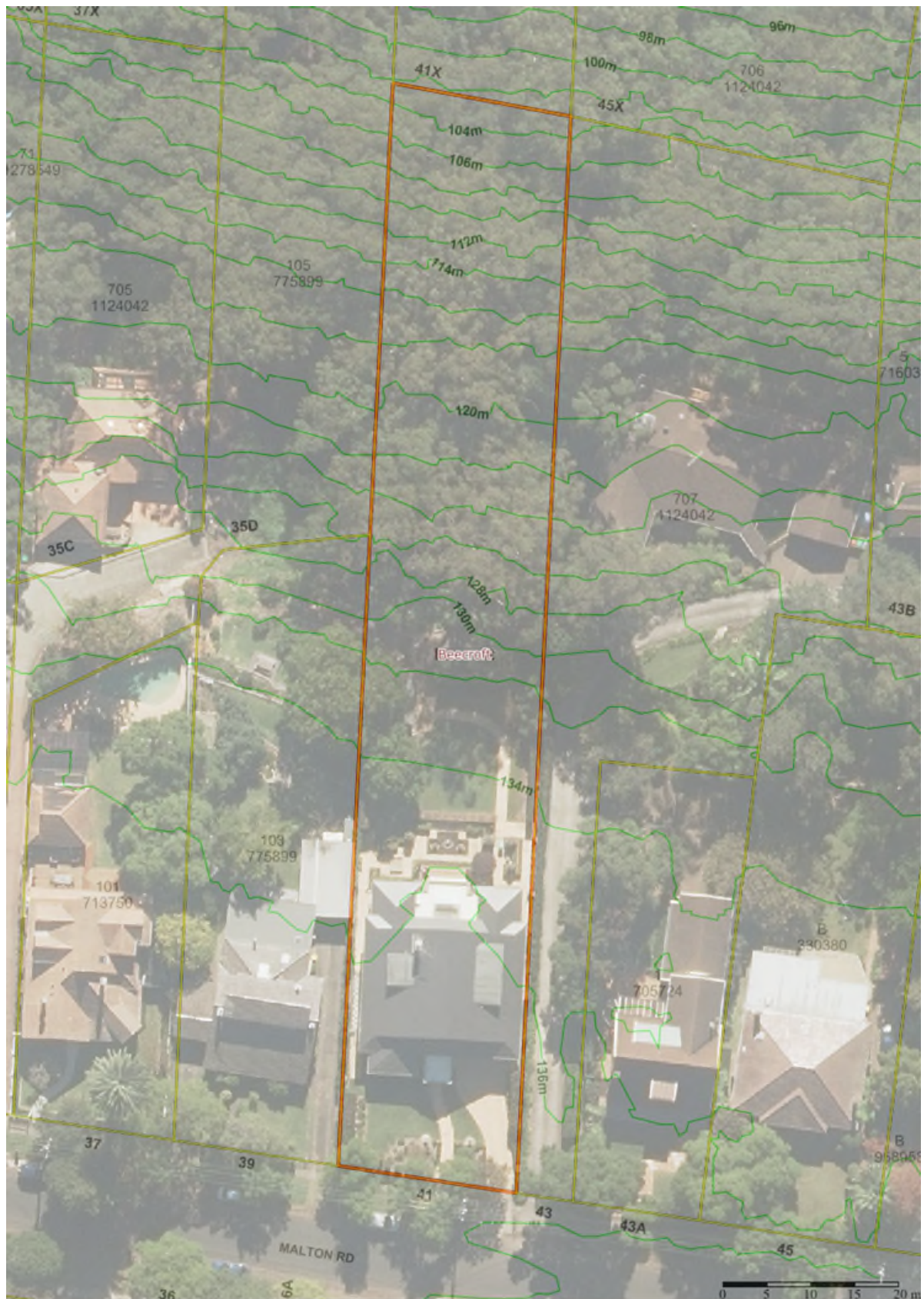
Figure 12: Aerial image of No. 41 Malton Road, Beecroft
