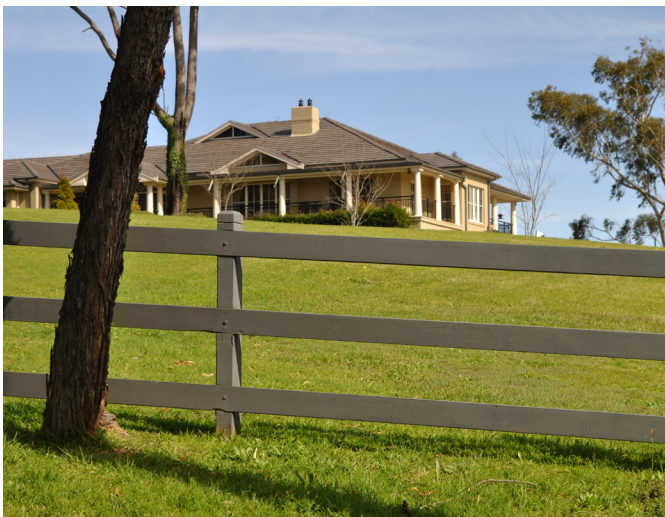
Figure 2.1(e): Example of a dwelling house designed and sited to contribute positively to the rural landscape. (E)
