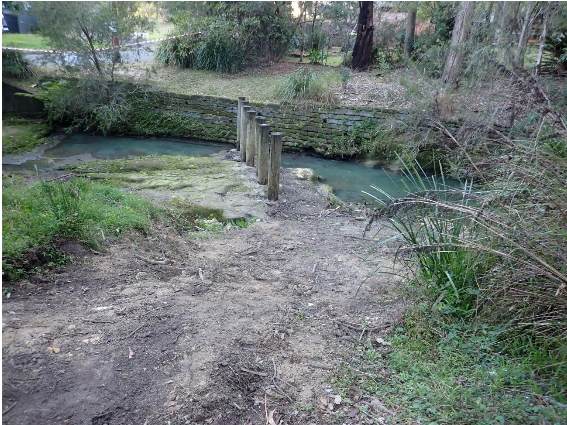
Figure 3 The site of the proposed GPT would be on the eastern side of Larool Creek behind a retaining wall
