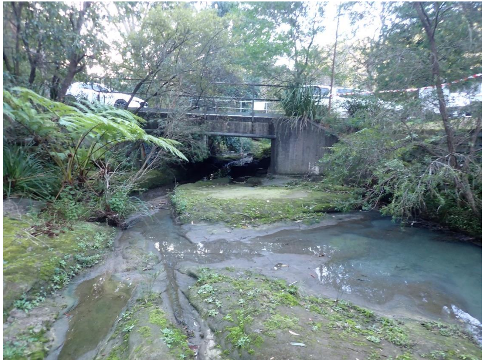
Figure 11 Downstream, the creek drains under Derribong Place via a concrete culvert
