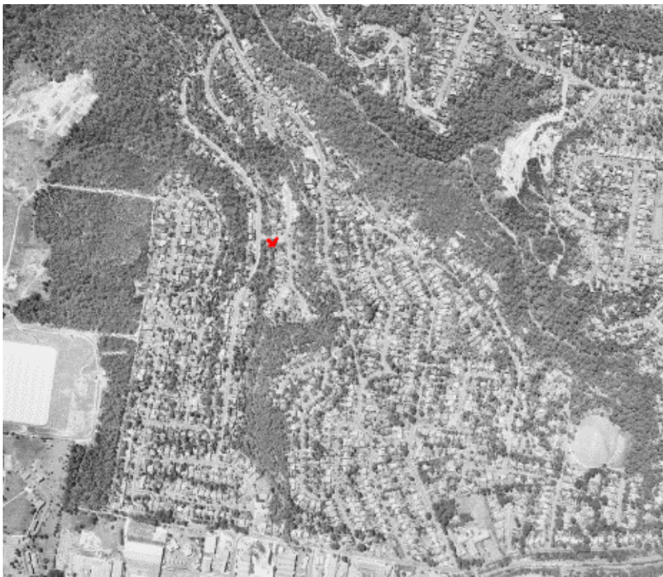
Figure 8 Aerial imagery from 1978 ( Historical Imagery (nsw.gov.au) ); Larool Creek catchment is fully developed
