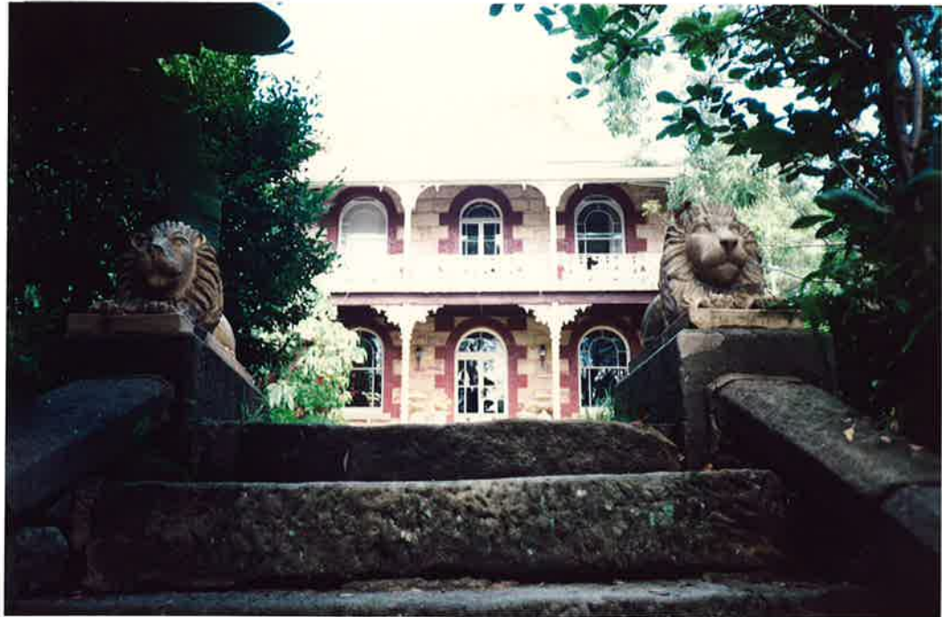
'Stanley House' 58 Pembroke Street Epping
