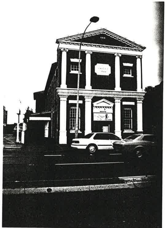
Masonic Hall 127 Pacific Highway Hornsby
