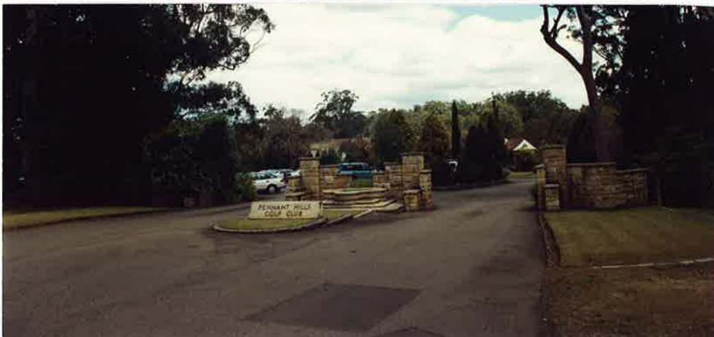
Pennant Hills Golf Club: Sandstone entry piers, c. 1950 (?).
