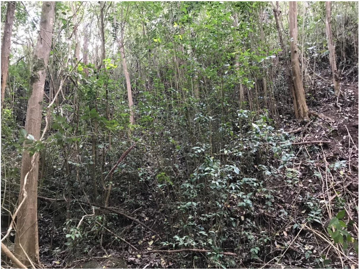
Photo Point 04 – MZ4 – Base of unstable mound to be removed - Privet habitat to be retained
