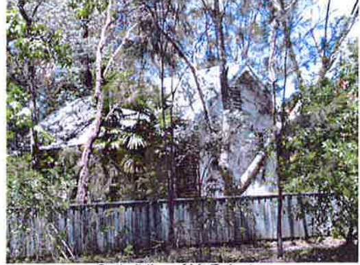
Outbuilding of Mt Errington
