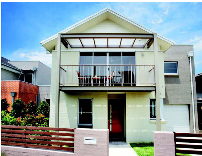
Figure 3.1(h): The main entry should be clearly visible from the street and sheltered from the weather, and the garages set back from the front facade. (E)
