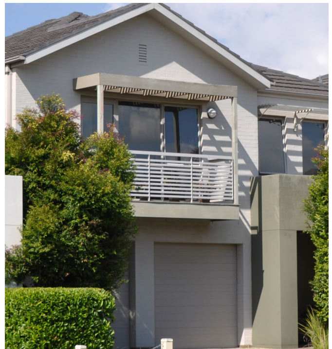
Figure 3.1(f): Sun shading devices are essential elements of a well designed home.(E)
