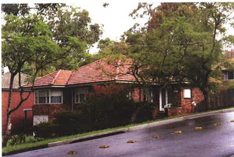
Figure 3.7 Good quality Post-War brick and tile single-storey house.
