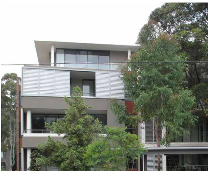
Figure 3.4(c): Desirable features- top storey set back with wide eaves (no parapets).(E)
