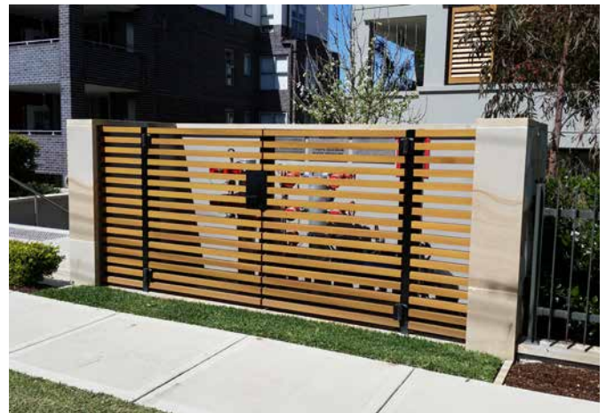
Figure 3.4(j): Example of the preferred style of screening for fire hydrants. Note: Screening must be designed to comply with AS 2419.
