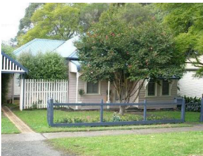
Figure 9.3(d): Take clues from traditional fences in the heritage conservation area. (E)
