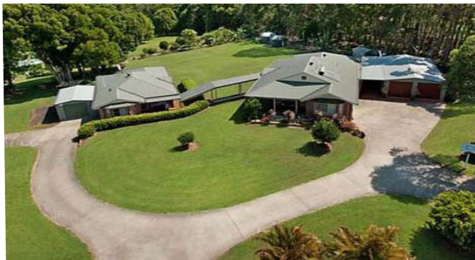
Figure 2.2(b): Covered walkways are not acceptable means of attaching the two dwellings. (E)
